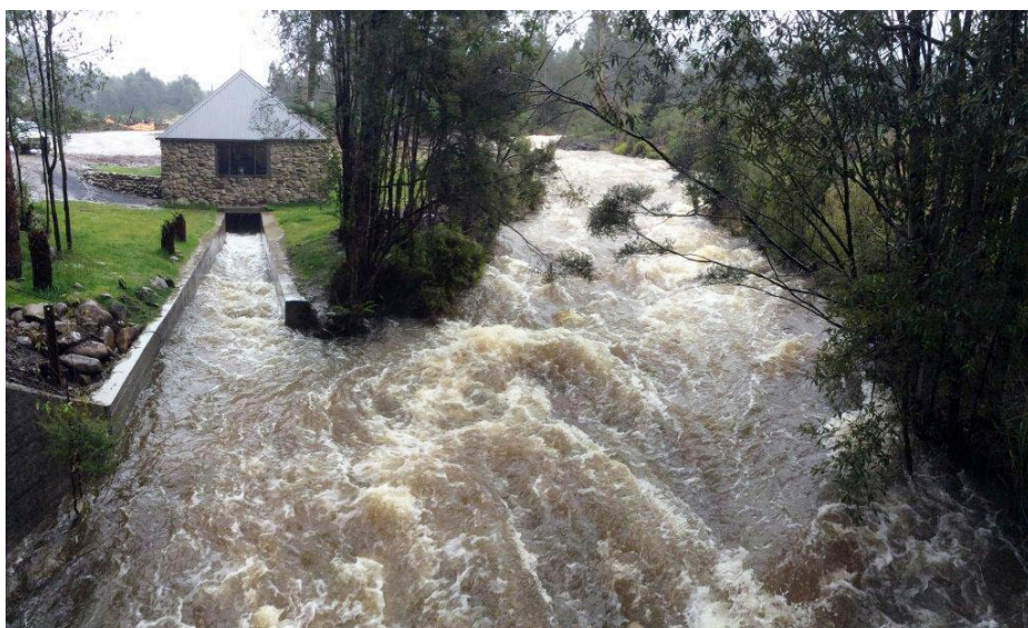
↑ Humboldt River power station and tailrace with the river in flood.
